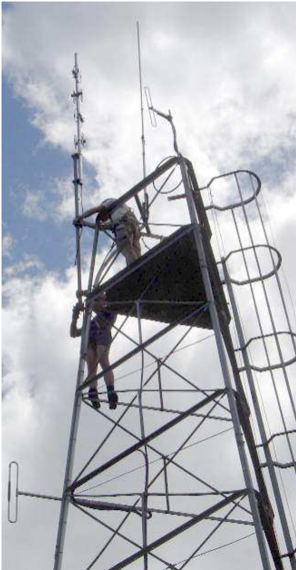
New 70cm antenna top left, 6m J-pole centre, and 2m antennas. 10m and 6m beacon antennas not visible to the right.
